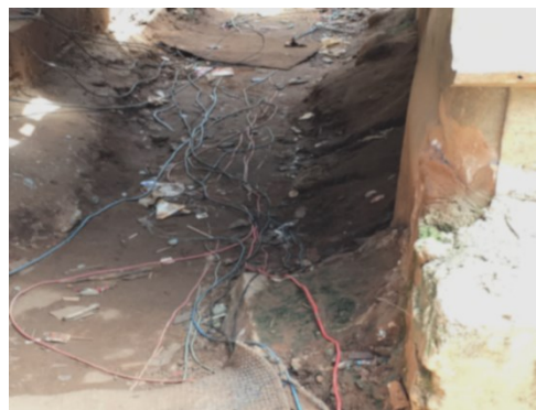
Figure 6. Example of live wires in Havelock.
